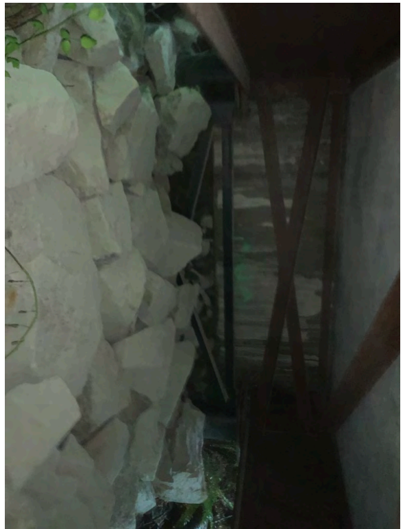
Right Bank Abutment when facing downstream
